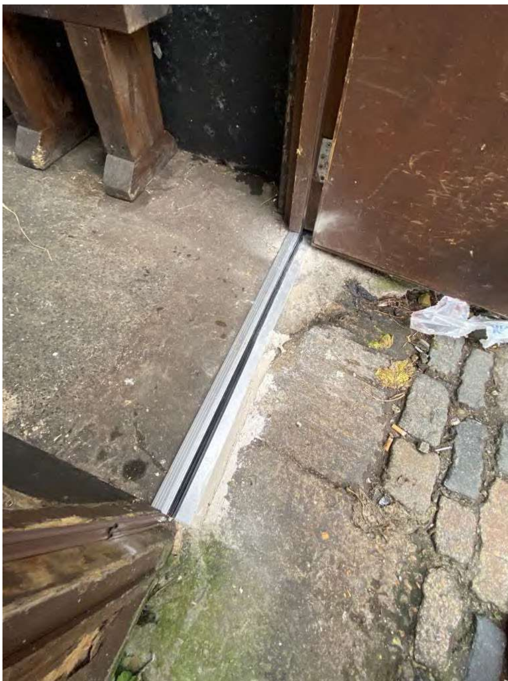
Figure 6: New threshold fitted to fire exit door
